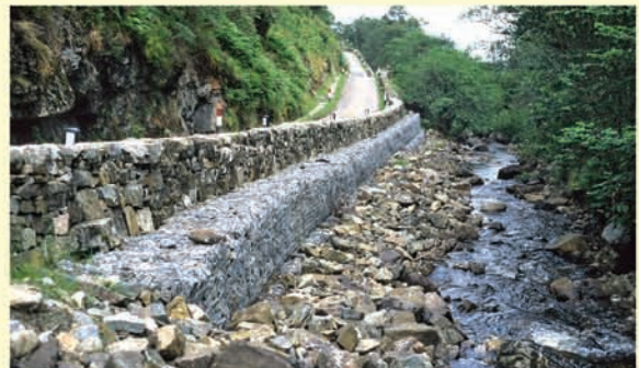
Gabion wall protecting a road from river erosion in Scotland.
