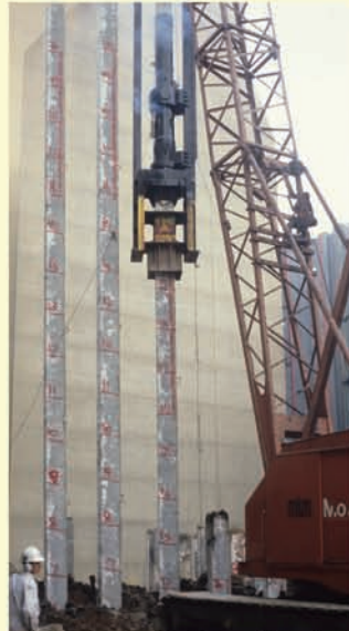
Driven piles in alluvial sand, England.
