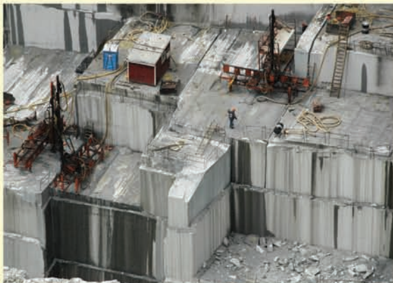
Faces cut by line drilling in granite, Rock of Ages quarry, Vermont.
