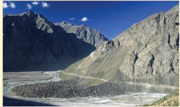
Road across scree and debris of large landslide, Indian Himalaya.
