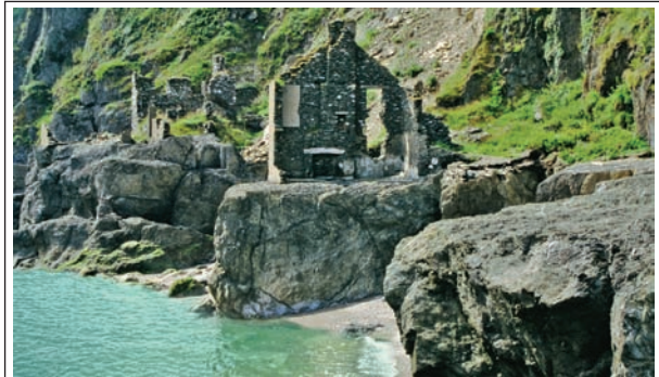
Hallsands village stood on a rock platform with a protective beach in front of it, on the Devon coast. In 1897, off-shore shingle dredging steepened the seabed sediment profile. Natural response was lowering and removal of beach within five years; so houses were exposed to waves, and destroyed in a storm in 1917.
