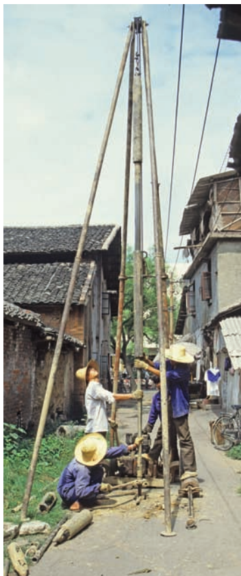
A traditional cable and tool rig in use in China, with its dropweight ready to fall onto the drill section.
