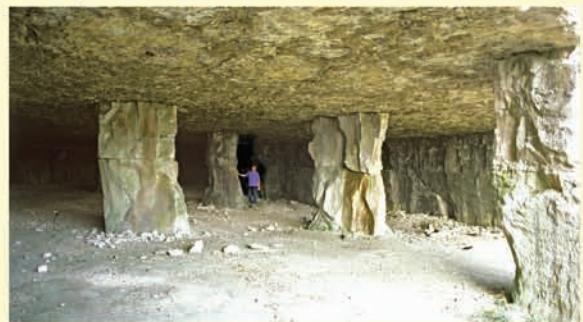
Old pillar-and-stall mine with thin pillars of strong limestone, Dorset.
