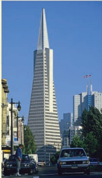
Earthquake-proof in San Francisco.
